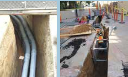
Deep trenches for conduits to carry electric lines
