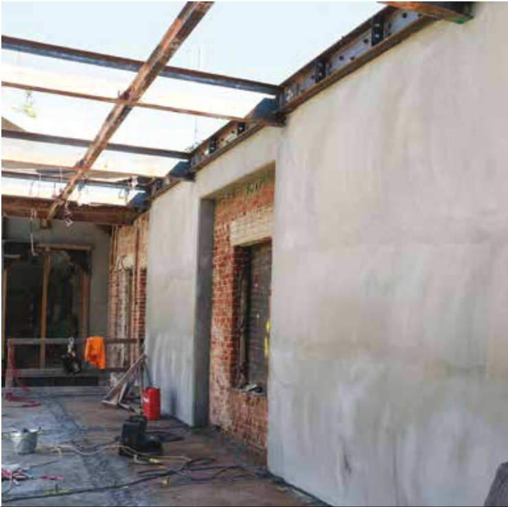
The finished walls on the upper level Post Office building after new shotcrete was applied.
