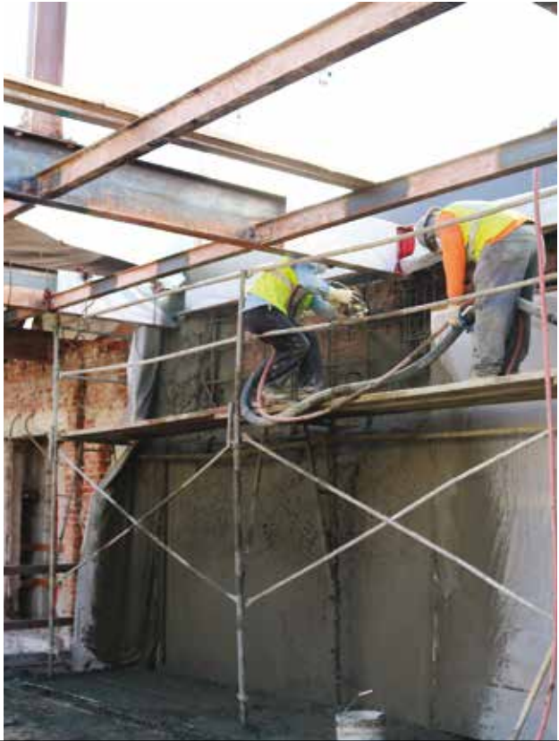
Workers apply shotcrete to the southerly wall of upper level Post Office building.
