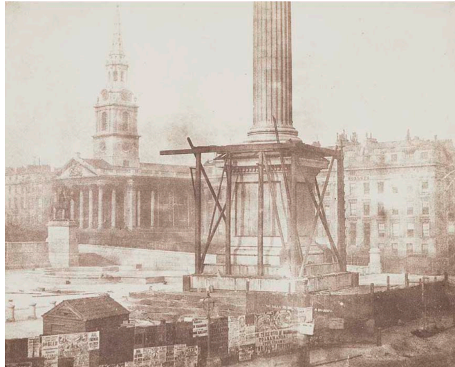
William Henry Fox Talbot, Nelson's Column under Construction, Trafalgar Square, London, first week of April 1844, printed later. Salted paper print. Courtesy of the Wilson Centre for Photography.
